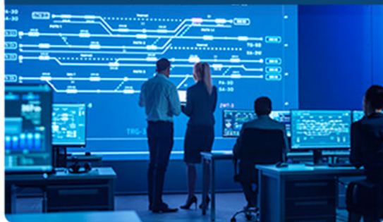
Transport Control Center
